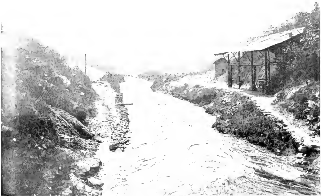
Pirahy Diversion: View down-stream from outlet of tunnel. Rio Light and Power Works.
